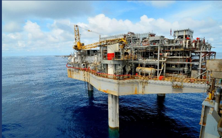
MOPU Production Equipment
